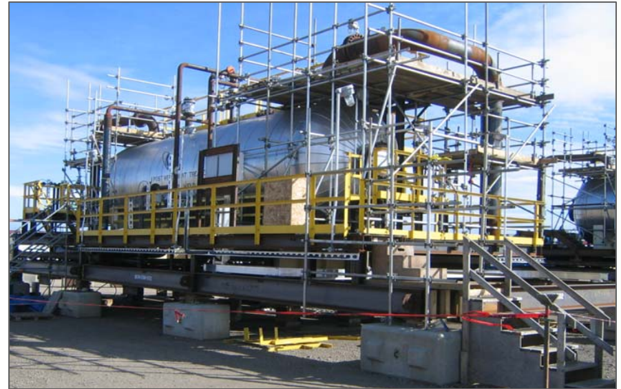
Photo: Modular fabrication of plant facility component
