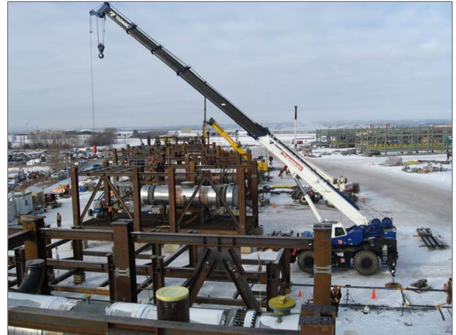
Photo: Fabrication yard in Sherwood Park
